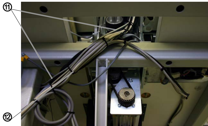
Fig. 11: Laying supply line B
