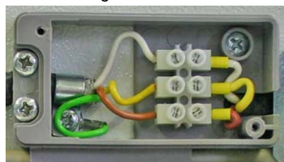
Figure. 36: Connecting the luster terminals
